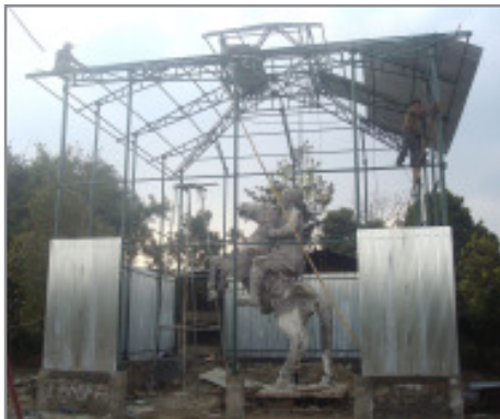
New workshop of SACH under construction.
