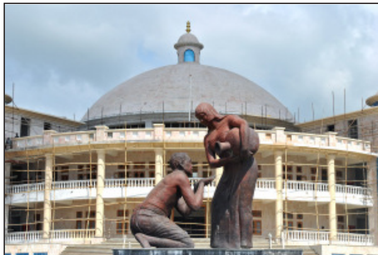
Sculpture in Bronze titled as 'Atithi Seva' developed and installed by SACH at the new Manipur Legislative Assembly complex, Chingmeirong, Imphal East.
