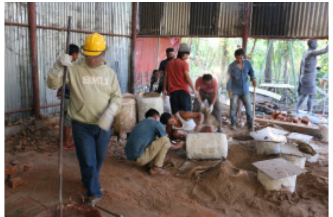
The team preparing for pouring
